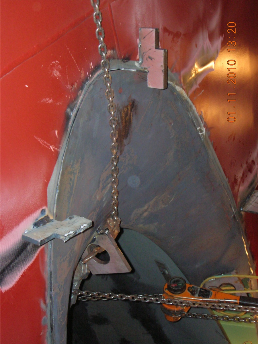
Casting attached on the hull.
